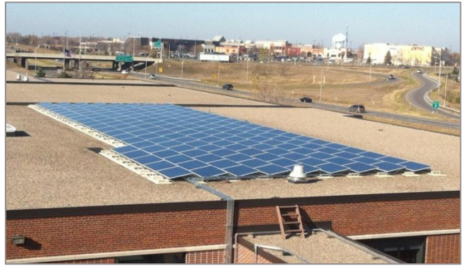
Minnesota Office Plaza, Roseville, MN. Photo courtesy of Solarflow
