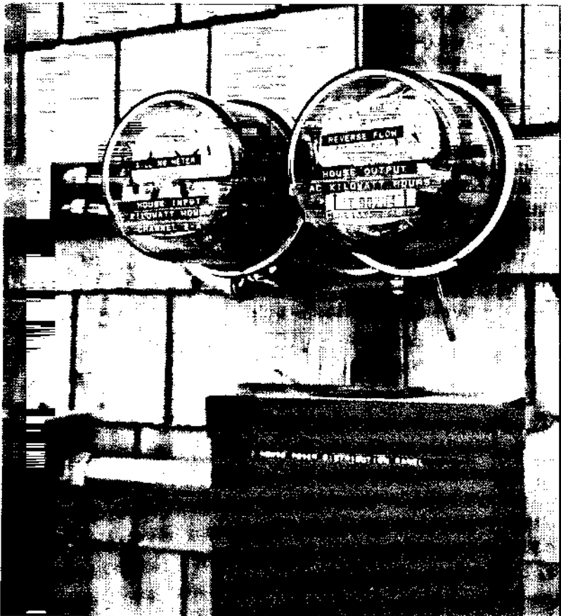
Photo 4-2: Shown here is a dual metering system. Reverse flow equals total wind system output to the grid (surplus overload), and the billing meter equals the total house load minus any wind system input to the house load. Photograph courtesy of Joe Carter.
