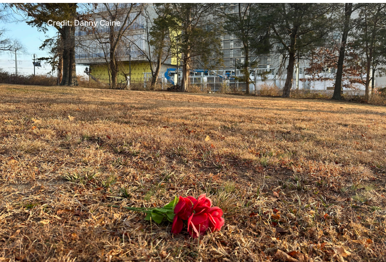
A hyperscale data center is under construction next to Tippett's Hill, a historic Black cemetery in Northern Virginia. "Nothing is sacred," said Elena Schlossberg, who has been deeply involved in organizing against data center development in the region.
