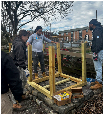
Compost bins under construction Credit: Philadelphia Parks and Recreation
