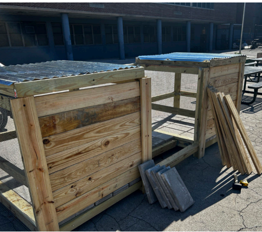
Compost bins under construction Credit: Philadelphia Parks and Recreation
