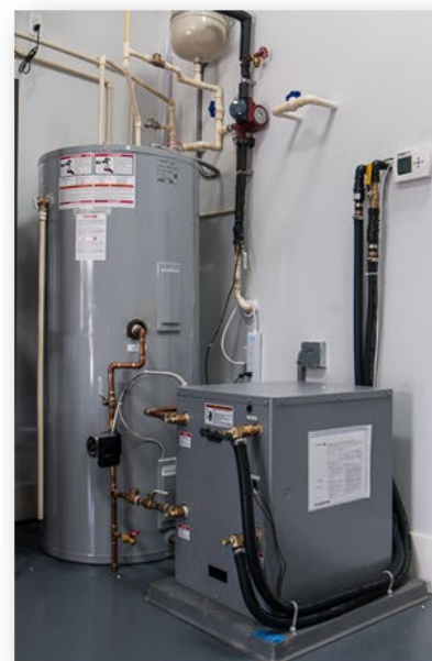
Dedicated Hot Water GHP (water-to-water GHP)
