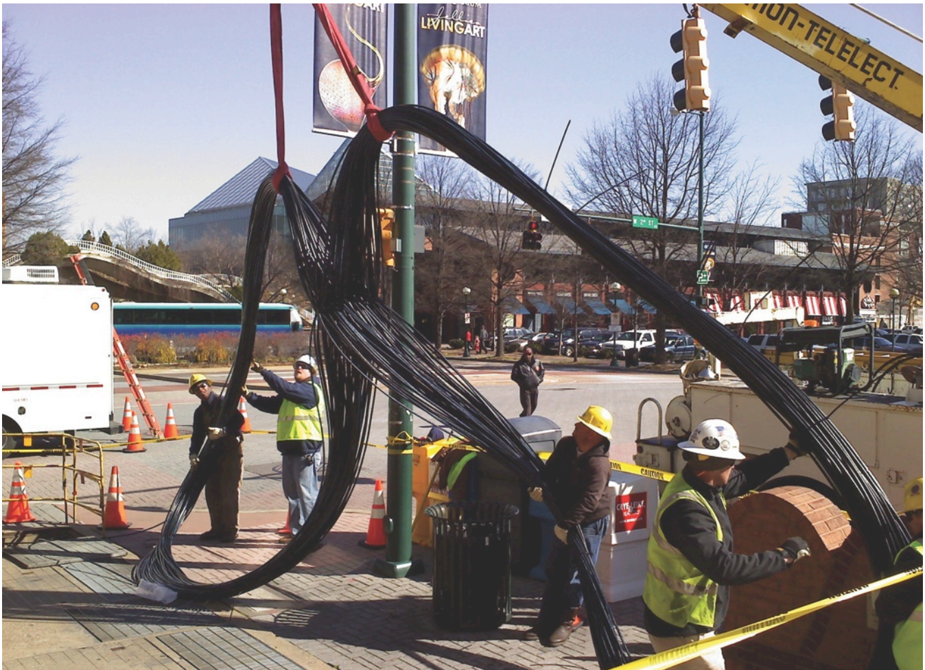
EPB Installs a lot of Fiber
