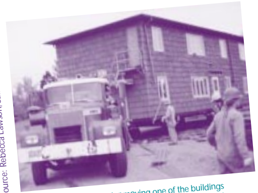
Contractor moving one of the buildings for the Bagley Downs apartment complex
